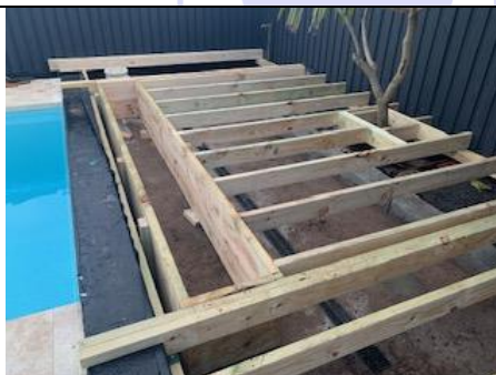
Cavity lining 190 x 35 or 245 x 35 as required
