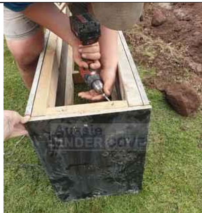
Screws must be accessible once the concrete has been poured so the form work can be removed
