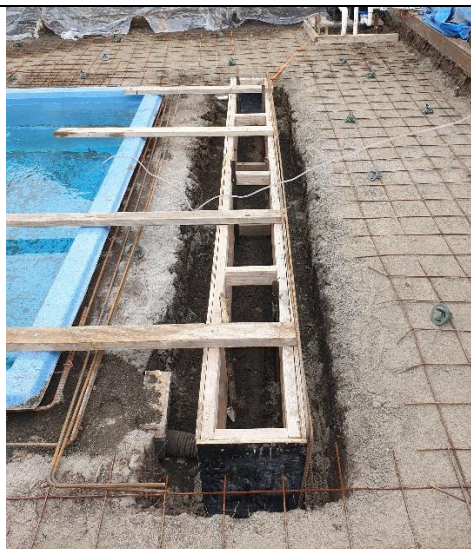
N12 rio in all walls & corners top and bottom Timber brace attached to formwork and pool edge to stop movement during concrete pour
