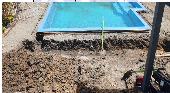
Completed form work 390mm wide x 500mm deep. Length to suit pool & kit
