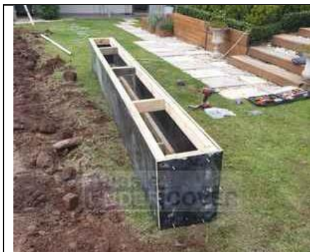
Overall completed formwork = Pit length by 400mm wide x 450/500mm high/deep
