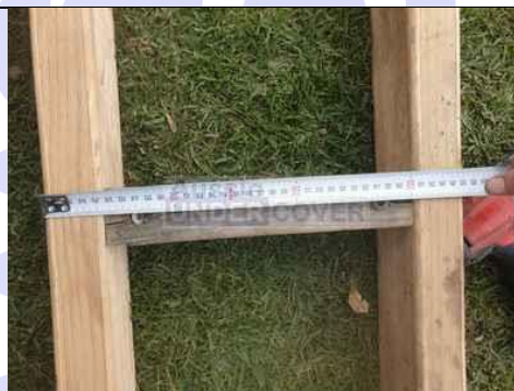
Outside to outside 360mm wide 90 x 45 treated pine. 20mm form ply will be added to each outside edge.
