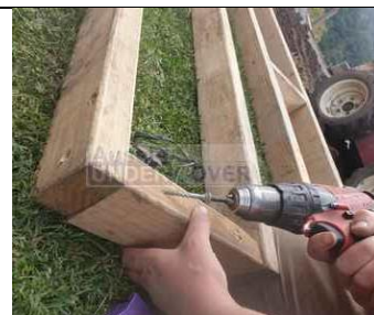
Screws must be accessible once the concrete has been poured so the form work can be removed
