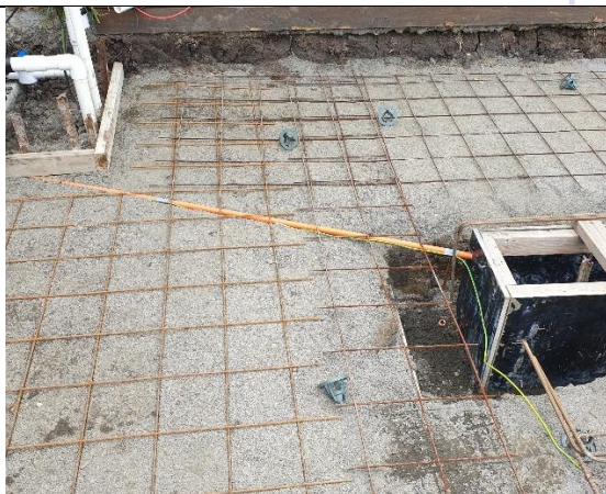
Conduit for power if required
