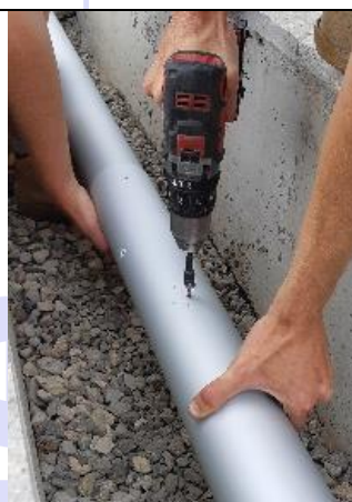
Secure tube joining screws
