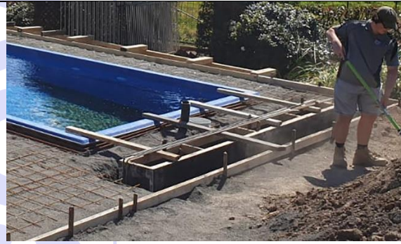
Pit formwork BRACED ready for concrete
