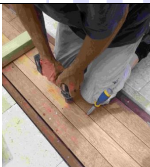
Screwing decking boards on Lid Frame
