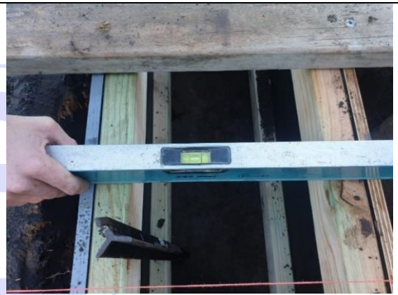
Figure 2 Ensure formwork is level horizontally and vertically
