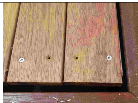
Pre-drill and countersink decking boards for lid
