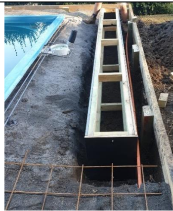
Figure 1 Form up concrete pit
