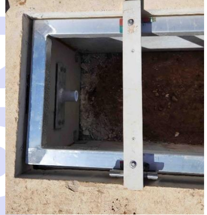
Support bracket ready for next hinge
