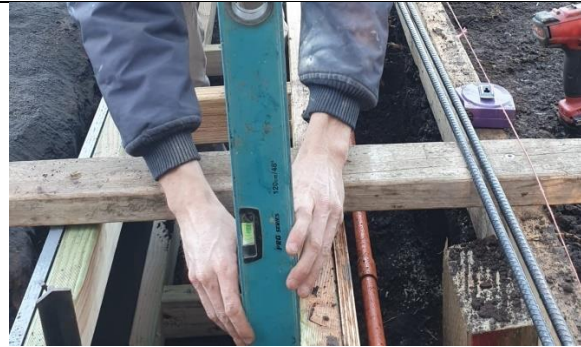
Figure 1 Form up concrete pit
