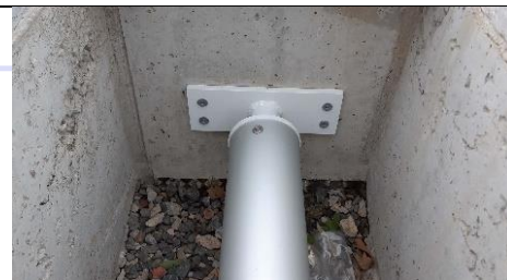
Insert the short End Slug into the End Mount
