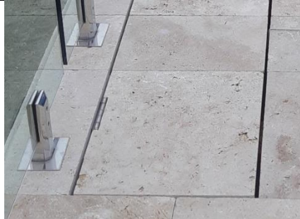
Cut tiles around hinges
