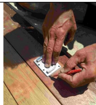
Marking handle position
