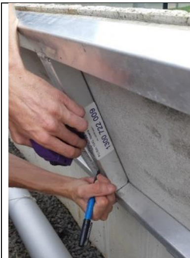
Mark 100mm to ball centre from bottom of lid frame
