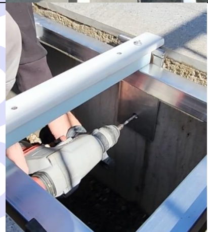
Predrill bottom of Hinge Plate
