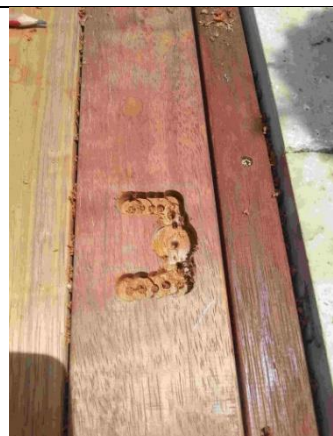
Completed drilling using speed bit
