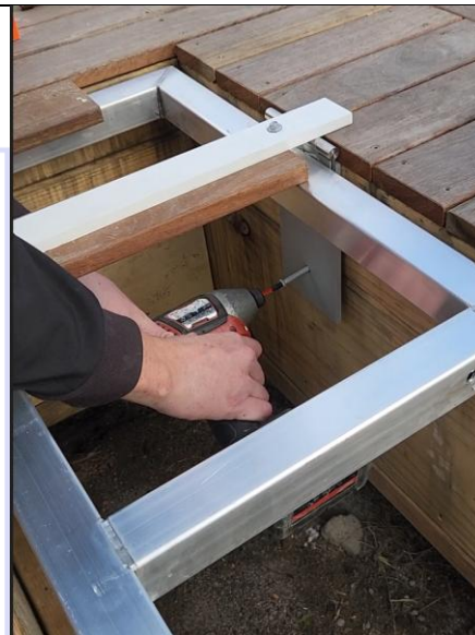
Predrill & screw bottom of Hinge Plate
