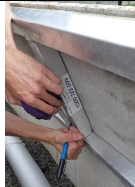
Mark 100mm to ball centre from bottom of lid frame
