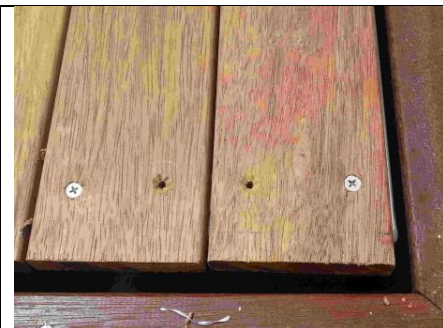
Pre-drill and countersink decking boards for lid
