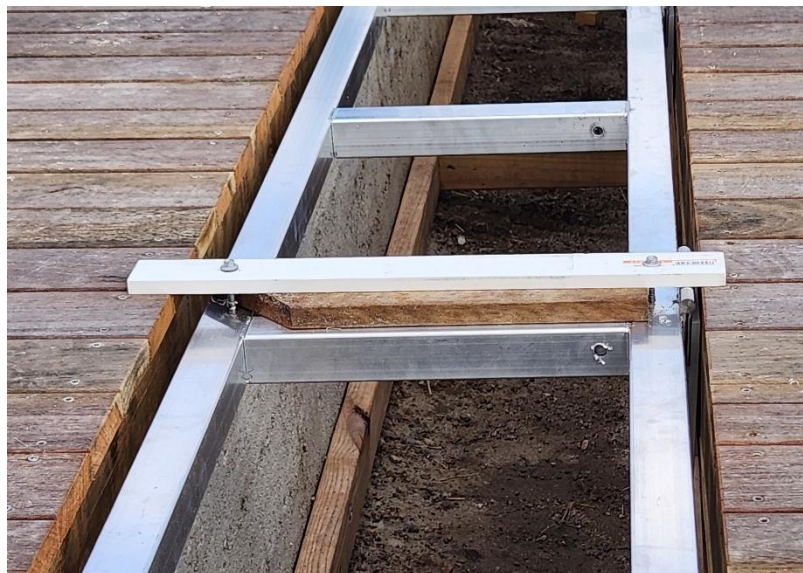
Ensure the Support bar is flush with both sides of the deck
