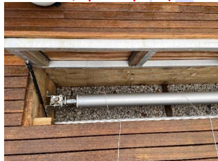
Timber 65 x 19 boards (6 boards)
