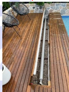
Timber 65 x 19 boards (6 boards)
