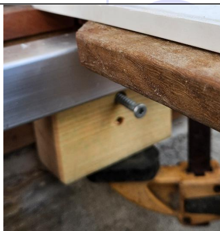
Position lid Block, redrill the existing hole if necessary
