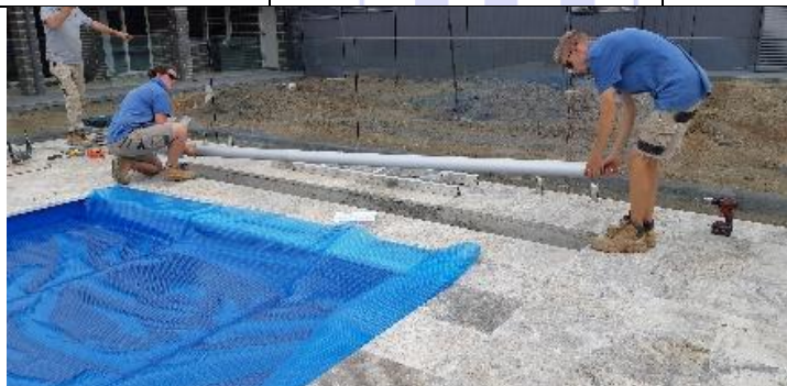
Install Small 95mm end slug
