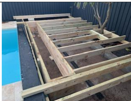
Cavity lining 190 x 35 or 245 x 35 as required
