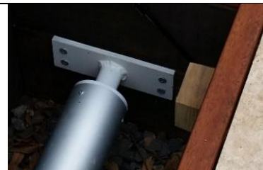
Insert the short End Slug into the End Mount
