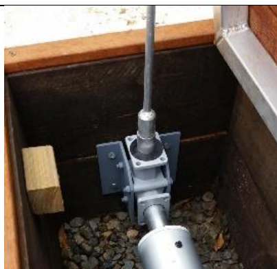
Insert tube assembly onto the end slug attached to the gearbox and screw in place
