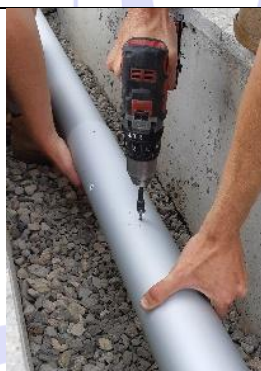
Secure tube joining screws
