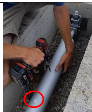
Install extra feather clips if necessary
