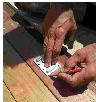
Marking handle position
