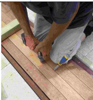
Screwing decking boards on Lid Frame
