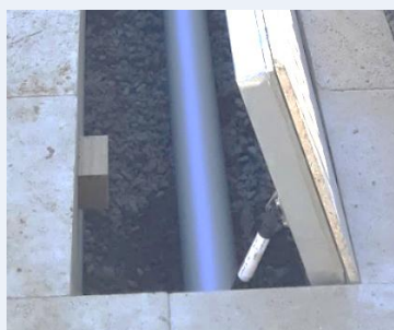
7.5mm Hardipanel and 12mm tile on lid frame
