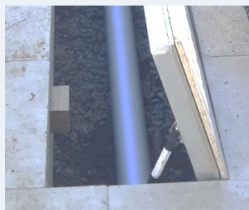
7.5mm Hardipanel and 12mm tile on lid frame
