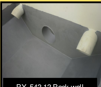
BX-543 13 Back wall blasted
