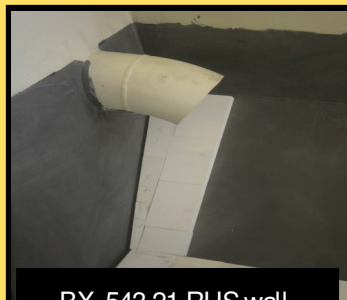
BX-543 21 RHS wall, marking out tiles ready for installation
