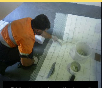
BX-543 26 Installation of floor & wall tiles
