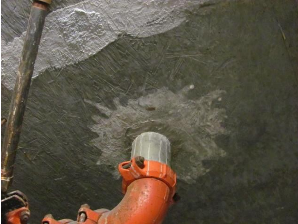
Repaired ceiling slab
