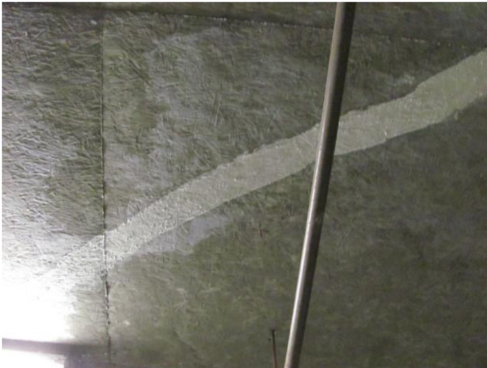
Repaired ceiling slab
