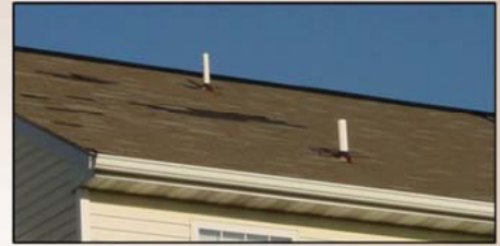
MISSING SHINGLES
