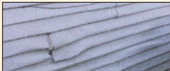
Melted Siding
