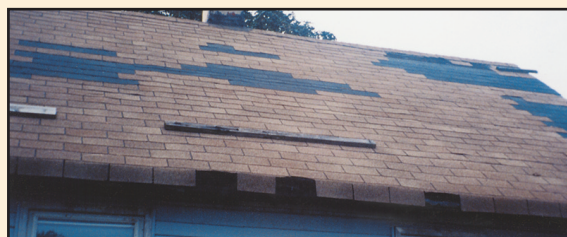
Missing Shingles
