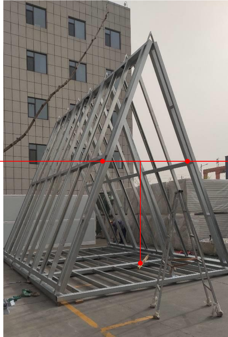
3 frame combinations (3 floor frames+6 roof frames)
