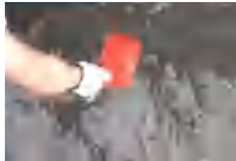
4. Apply Fresh Cement Slurry
