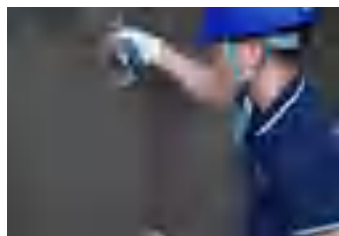
8. Apply Adhesive on Level Wall/ Floor
