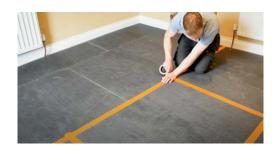
**4.** Tape over the butt joints to prevent any movement over time.
