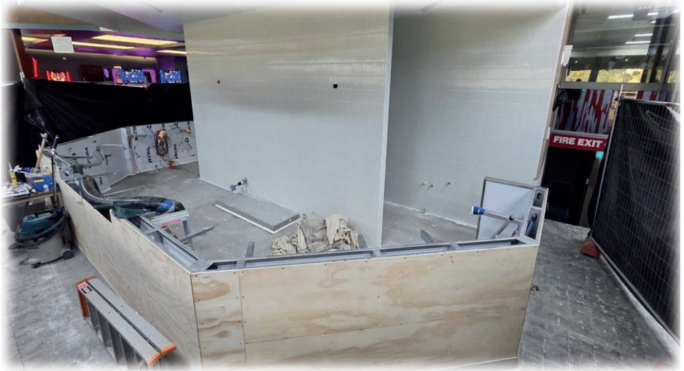
BELOW: The Club's main bar throughout the renovations.
