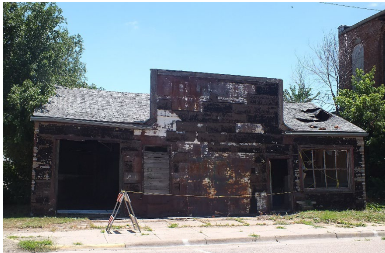
Street view of 406 S Orleans Ave 'shop building'.
