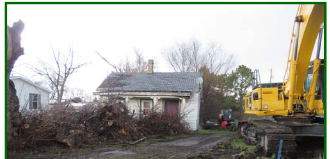
A dilapidated house being demolished in Axtell.
