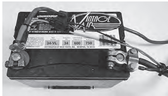
Completed Installation Shown
