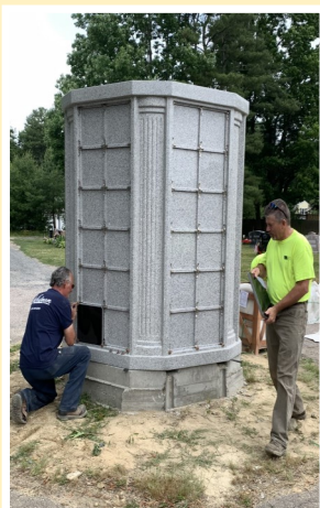
Our new columbarium being installed
