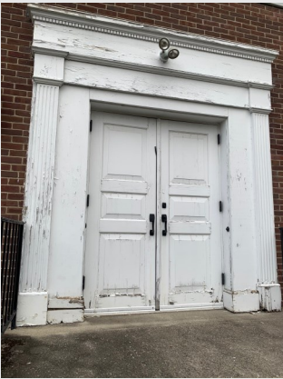
Chapel Doors (Before)
