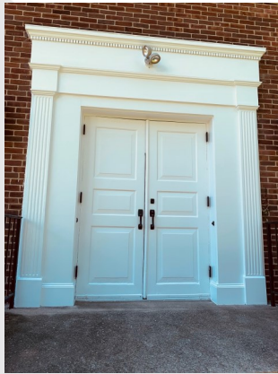
Chapel Doors (After)
