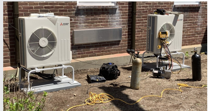
Installation of new AC units at St. Basil's Chapel
