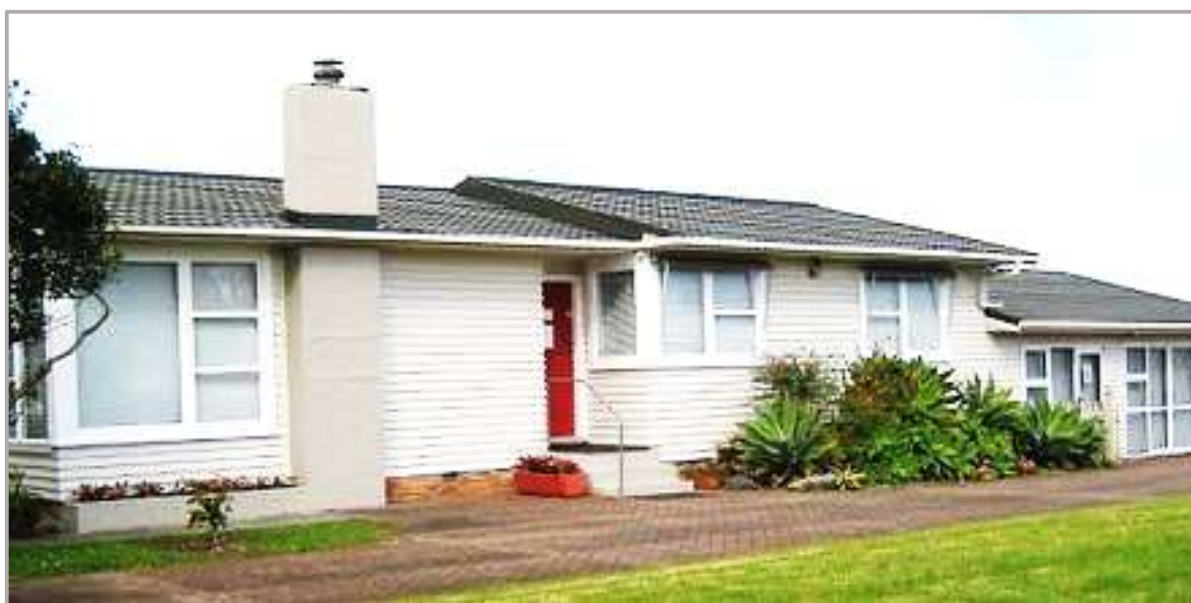
PCC in 2012 after conversion and a new roof
