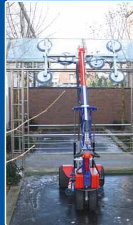
An especially long telescopic on installation on a height of 3 m.
