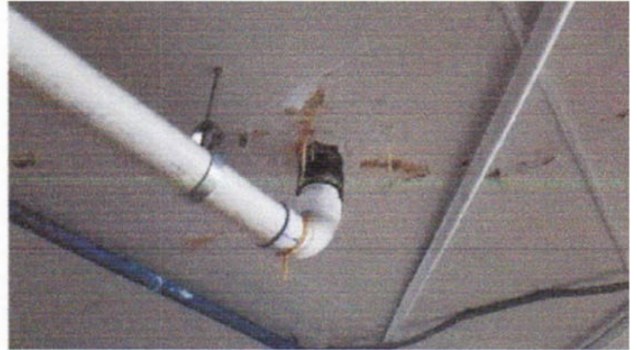
Figure K1: Previously installed failed injection repairs with leaching forming
