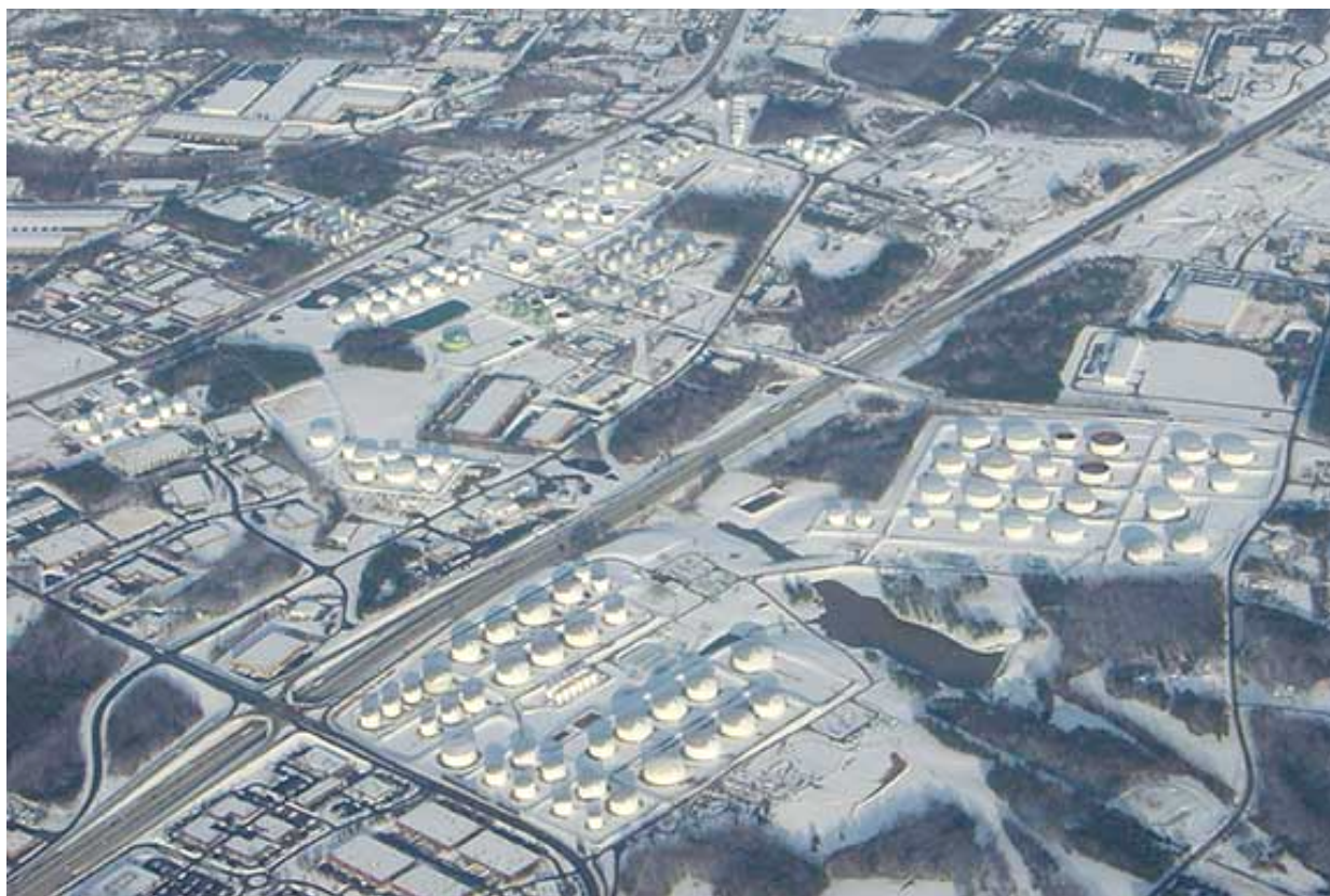
The author snapped this photo of the 73-tanks of the Colonial Pipeline tank farm in Greensboro, NC one winter day a couple of years ago. This node on the huge Colonial network moves about 18% of all the petroleum products used in the US on any given day safely and quickly. The small size of the market for avgas means it cannot use any of these efficiencies.
