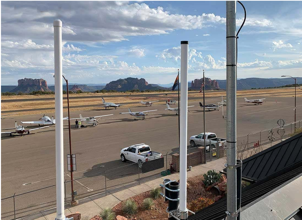
Photo 1: Unlike other airplane tracking systems, VirTower installs a small but powerful ground system on the premises of each customer airport (the two white antennae). These are linked to the internet and a giant cloud computing system which makes real-time tracking possible, and the analysis of the collected data quick, easy and reliable. All the airport needs to provide is a bit of electricity and a tall rooftop.
