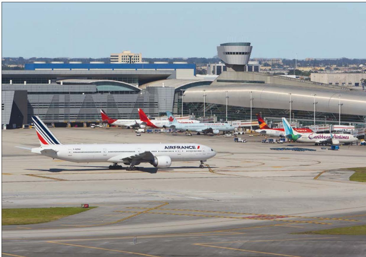
Crews work around the clock to inspect the vast expanse of paved airfield at MIA.
