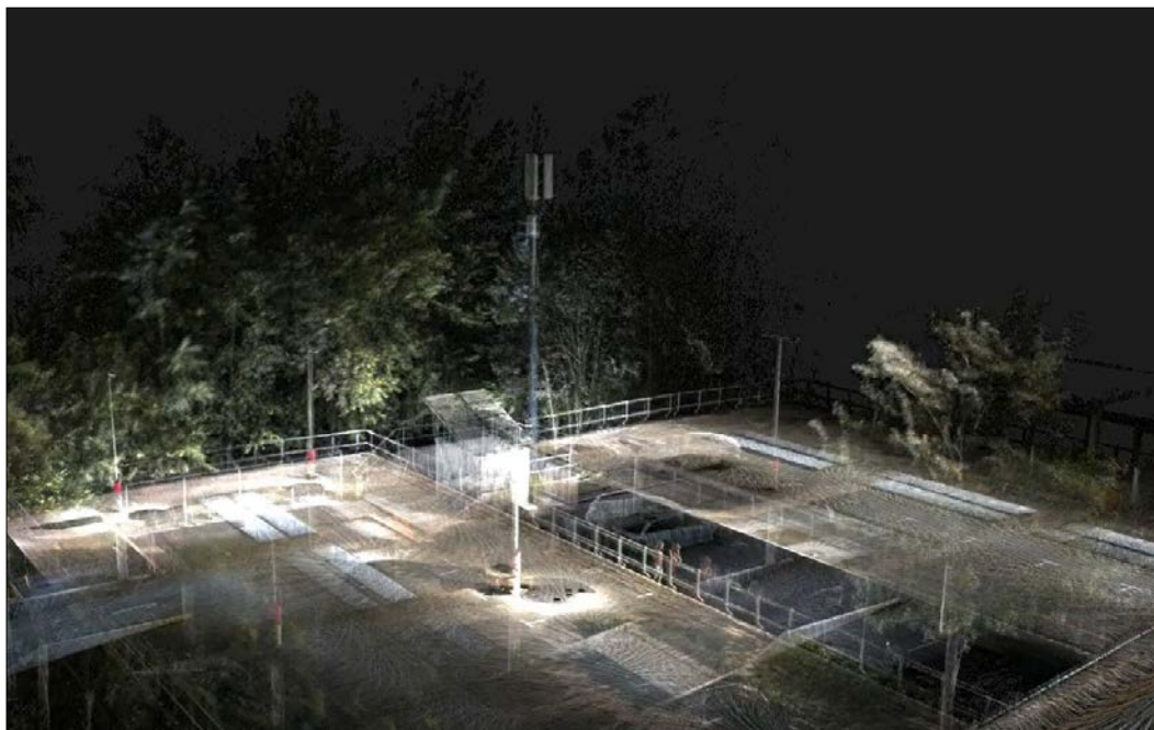
The digital twin captures some things at higher levels of detail than others, such as this cell tower captured along with the complex urban environment around it. Image courtesy of Vodafone.
