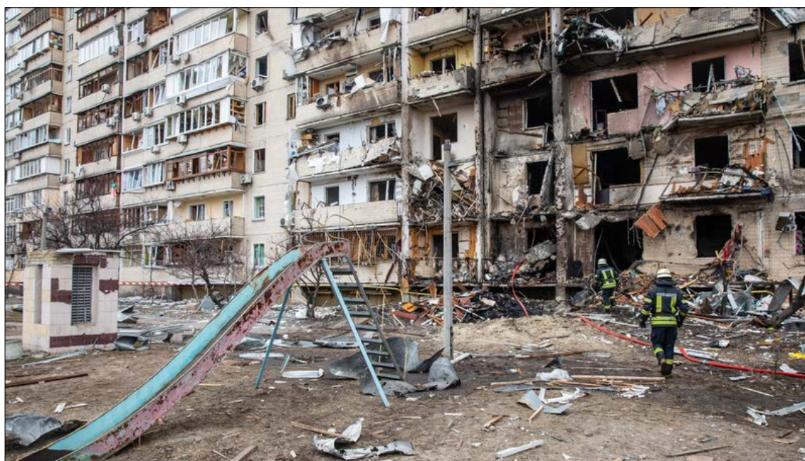
Much of the destruction in Ukraine surrounds civilian areas, such as this damaged apartment building in Kyiv.
