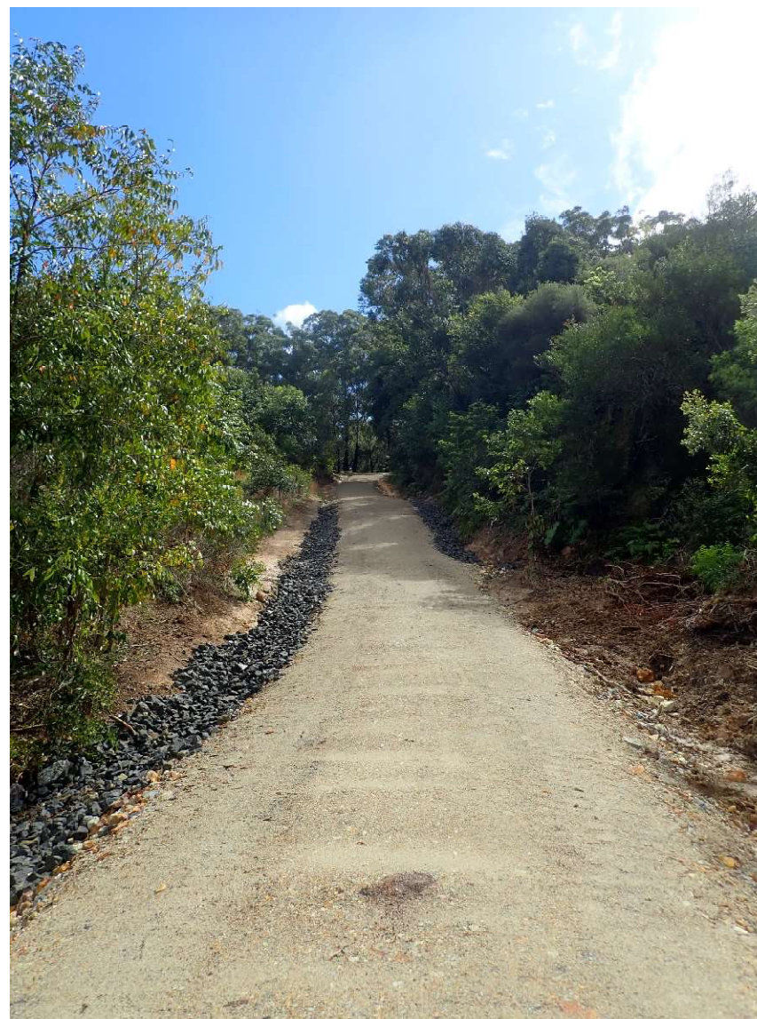
Picture 33 (looking down road) & 34 (looking up road) – Repaired road and edge drain
