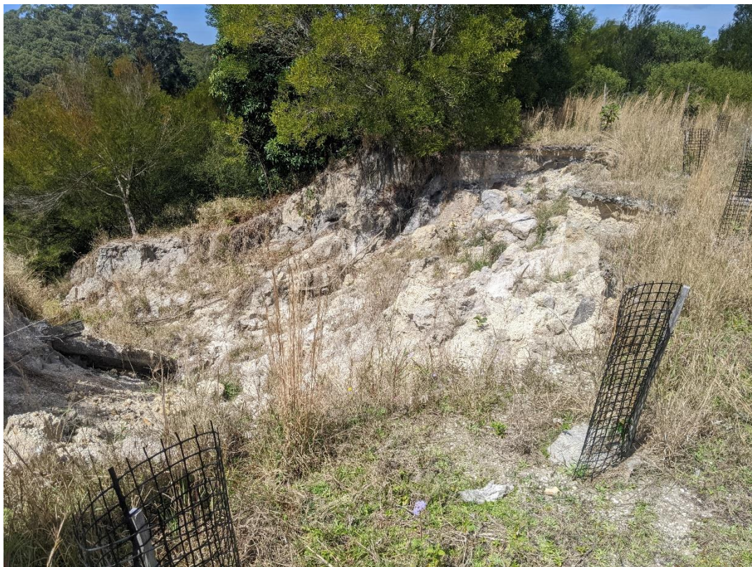
Photo 4 – This area requires repair. Significant mass movement needs to be reshaped and stabilised. Upslope water needs to be diverted or directed downslope.
