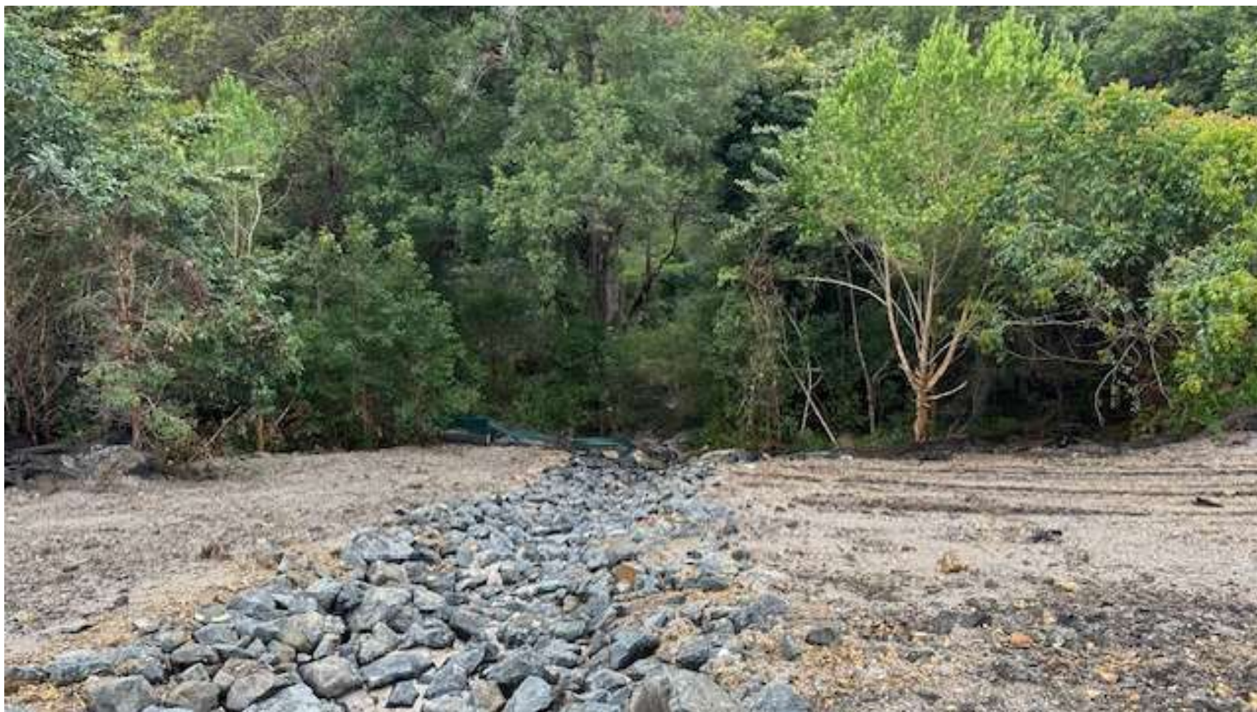
Picture 4 – new drain from culvert to detention basin
