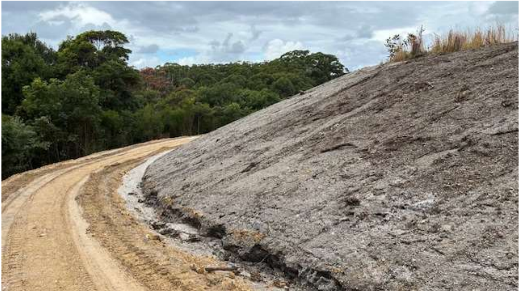
Picture 2 – extended batter remediation uphill of landslip, road edge drain
