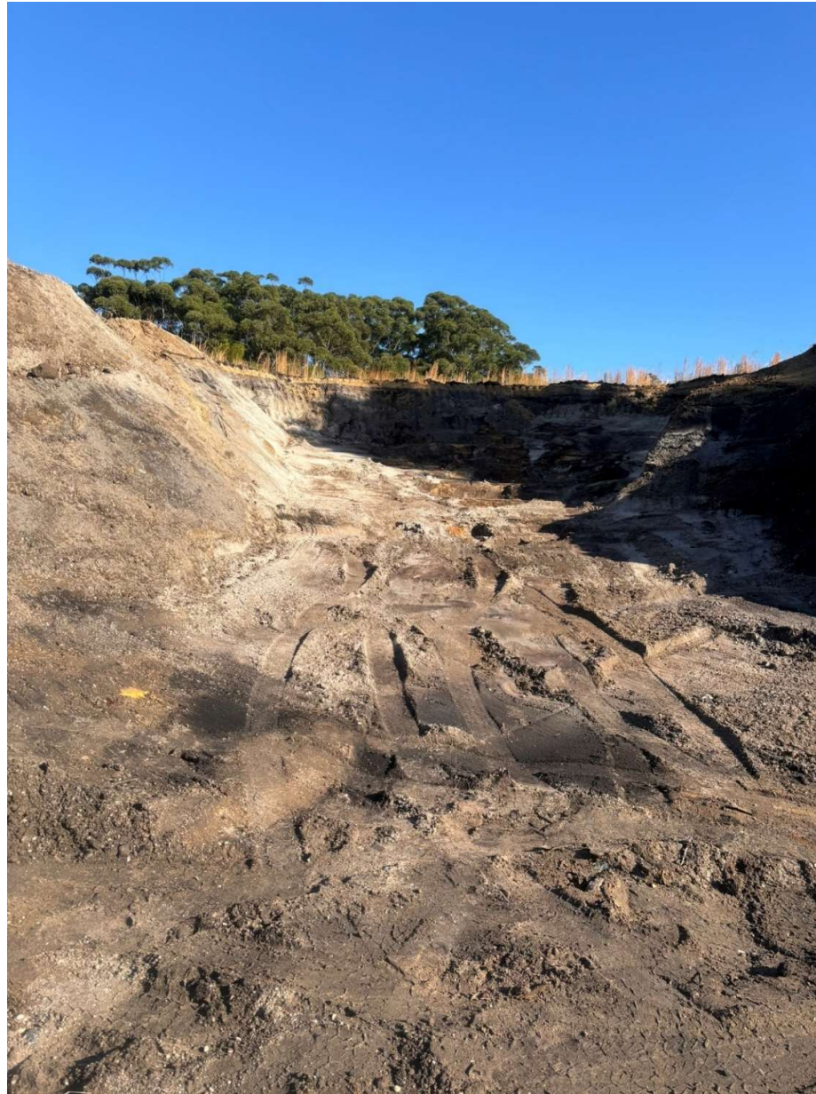
Picture 6 – original landslide location after vegetation clearance prior to reforming batter
