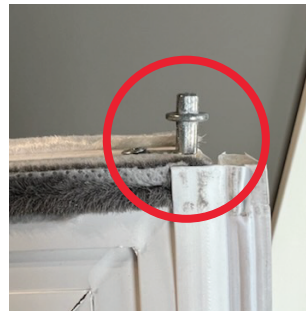
Double Hung (DH) Sash Pin
