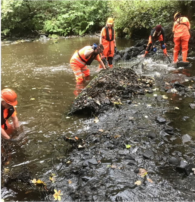
Dismantling the Gabion Weir
