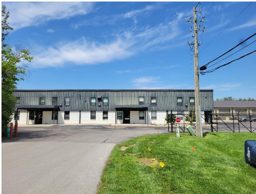
Photo 2: Adjacent Industrial Use to North
