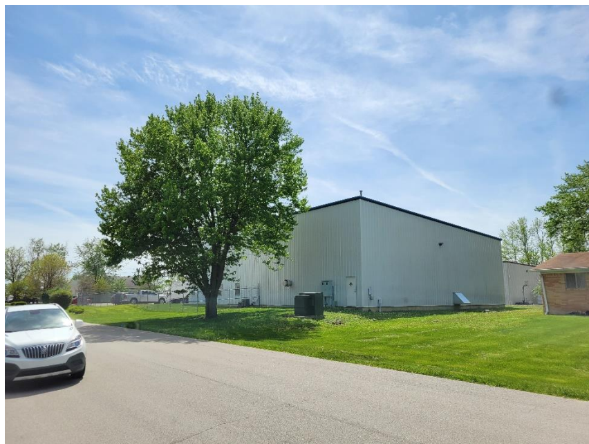
Photo 6: Adjacent Property to Southwest
