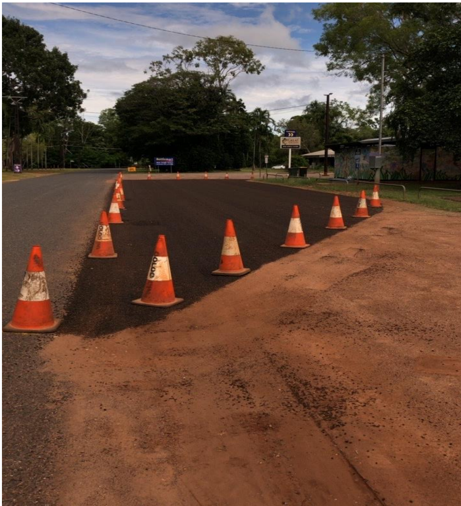
Sealing the Black Water Dump Point in Batchelor – April 2020
