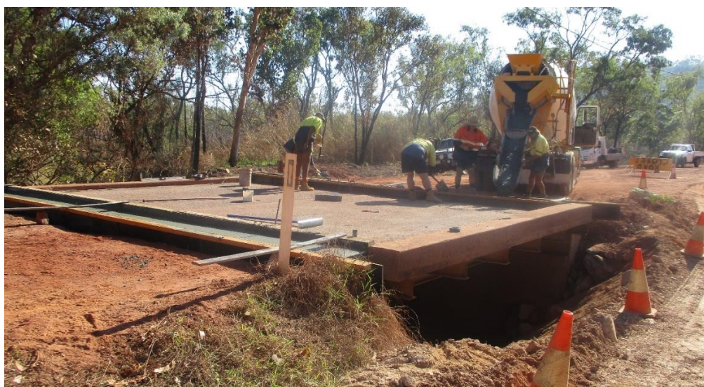
Coach Road Floodway – July 2019
