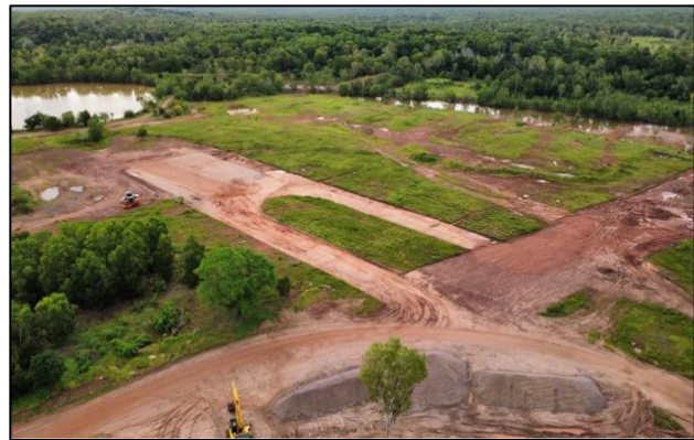
PREPARATIONS GROUNDWATER TREATMENT PLANT
