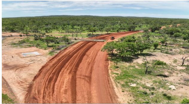
HAUL ROAD PROGRESSION
