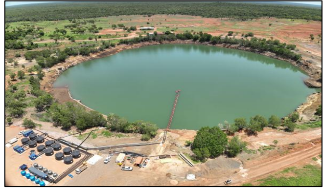
MAIN PIT THAT IS GETTING DEWATERED
