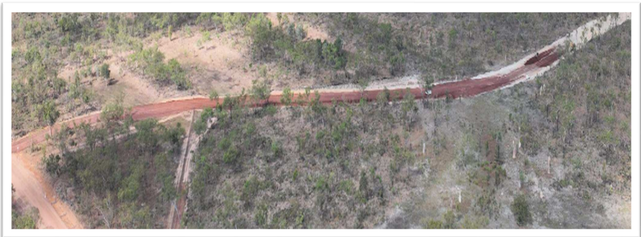
800 metre corridor of the A9 Haul Road crossing the FRALT toward construction material source
