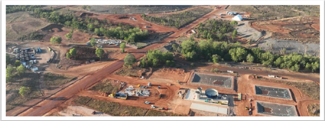
Stage 2 haul road, PWTP and workshop facilities in the foreground
