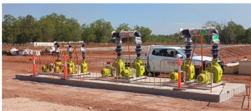
Ground Water Treatment Plant construction
