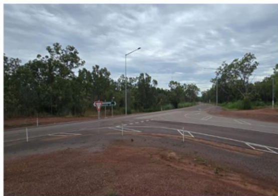
Poet Road and Litchfield Park Road Intersection upgrade.
