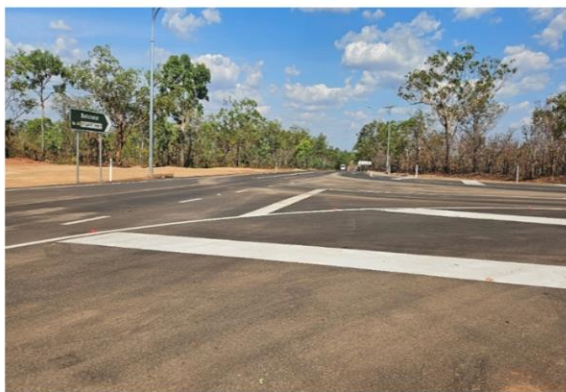
Batchelor Road and Litchfield Park Road Intersection
