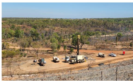
Ground water bore installation
