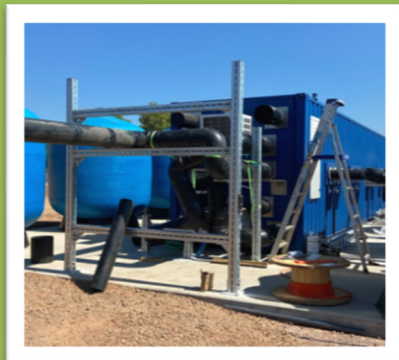
Filtration vessels and prefabricated piping manifold container
