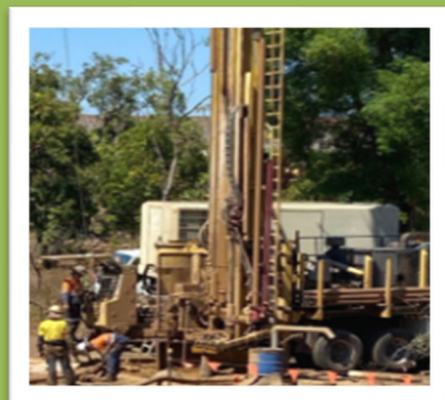
Crew undertaking ground water bore installation
