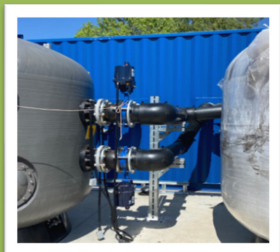
Filtration vessels and prefabricated piping manifold container
