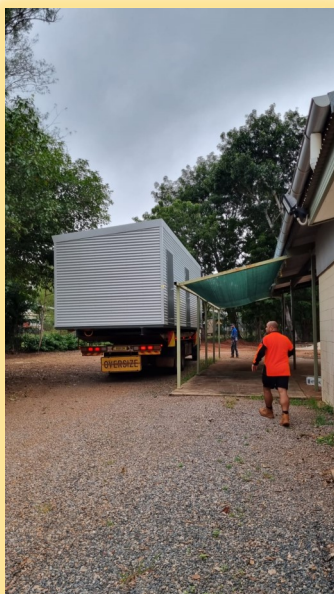
Delivery and Installation of the new ablution block at the Batchelor Office, Feb 2023.
