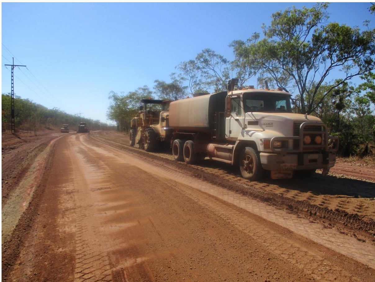
Gravelling and Sealing Coach Road – SLGIF and Roads to Recovery Grants
