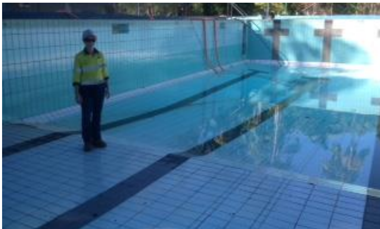
Batchelor Swimming Pool empty prior to upgrades – June 2018
