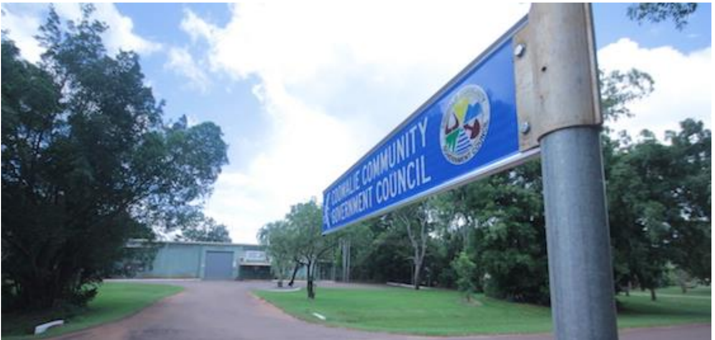
Council's Administration and Depot buildings
