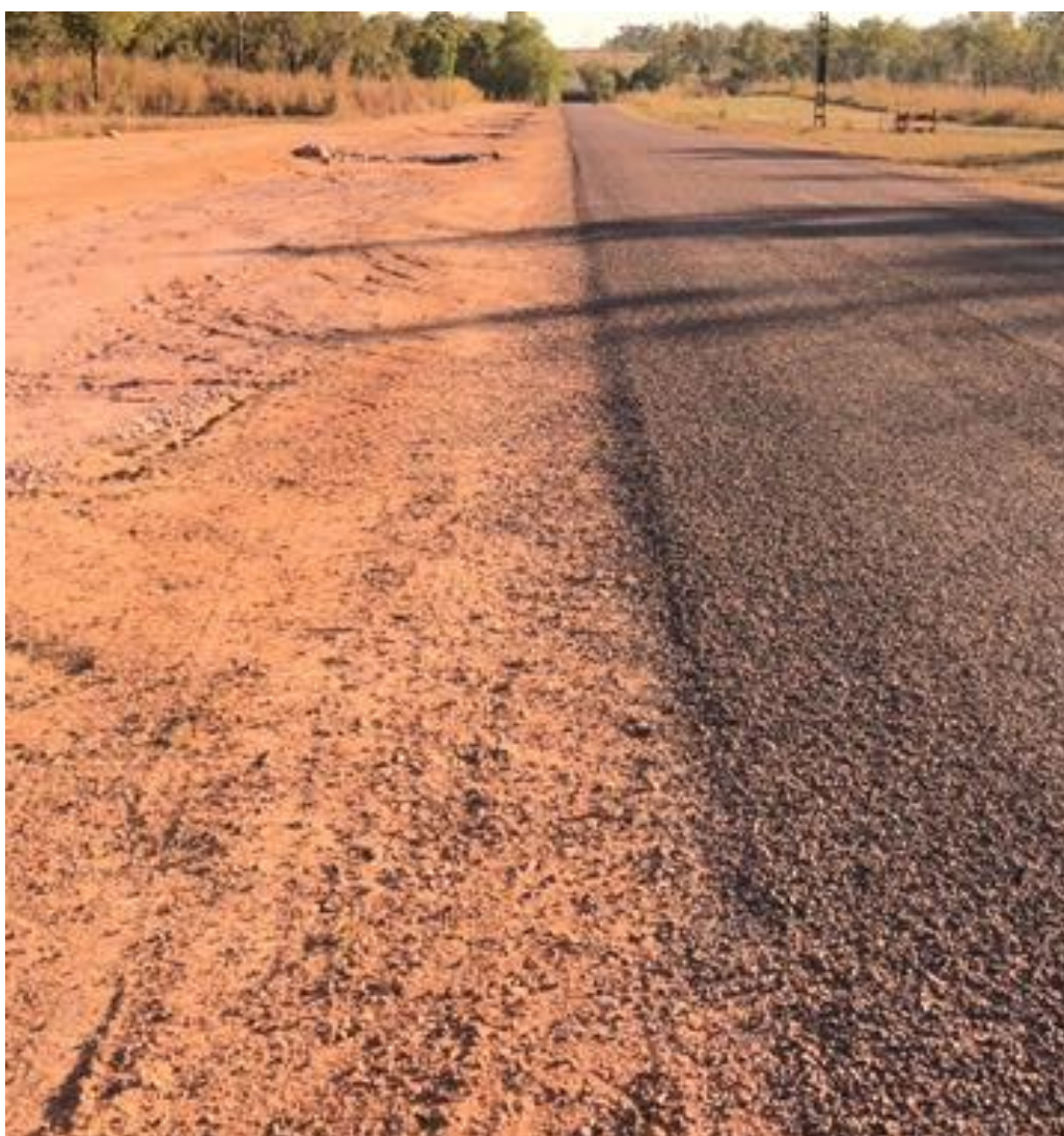
Flood Damage Repairs NDRRA Grant – Cheeney Road
