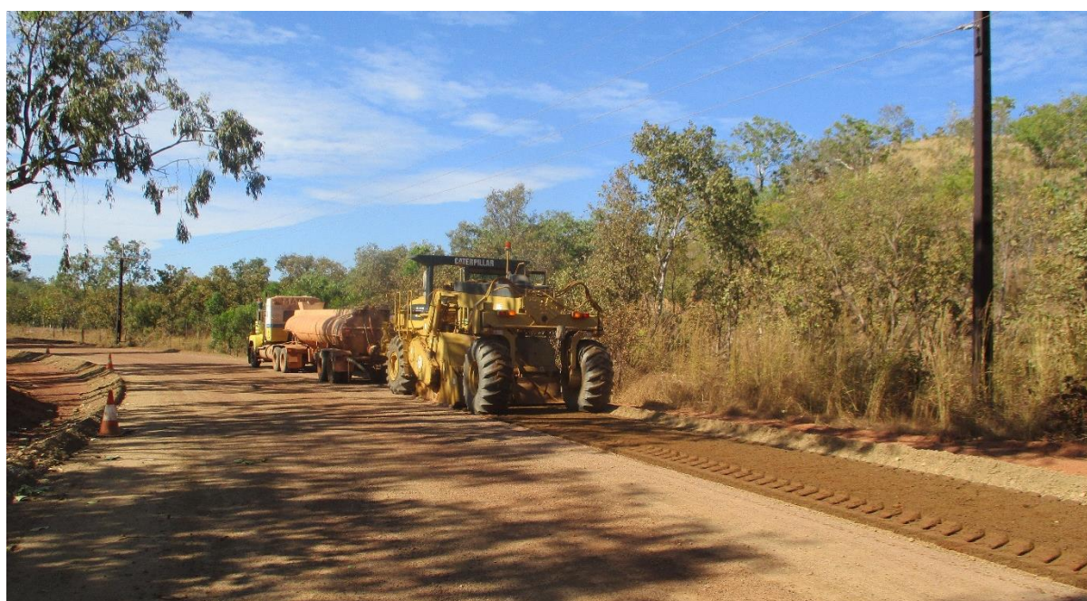
Gravelling and Sealing Coach Road – SLGIF and Roads to Recovery Grants
