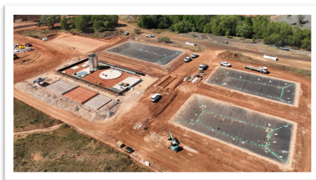
Groundwater treatment plant foundations
