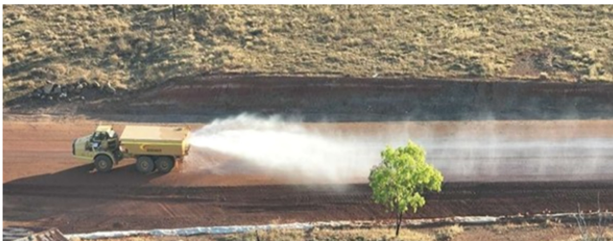
Haul road maintenance (dust suppression)
