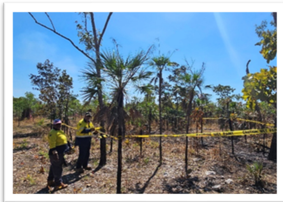
Land Management Team members pegging and flagging the A9 haul road alignment
