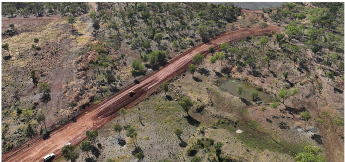
Haul road construction towards Dysons (Backfilled) Pit
