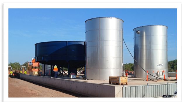
Groundwater treatment plant construction
