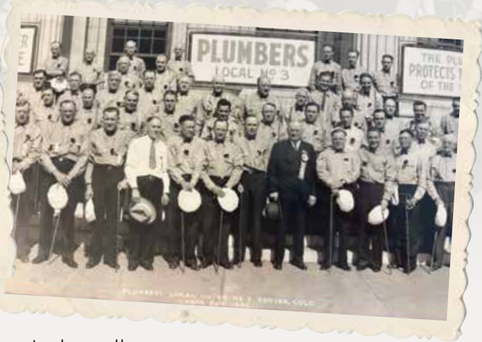
Val Palmer and Harold Christiansen stand outside their first office in Salt Lake in the 1940s (left); Local No. 3 union plumbers from the 1940s. (all photos courtesy Palmer-Christiansen)
