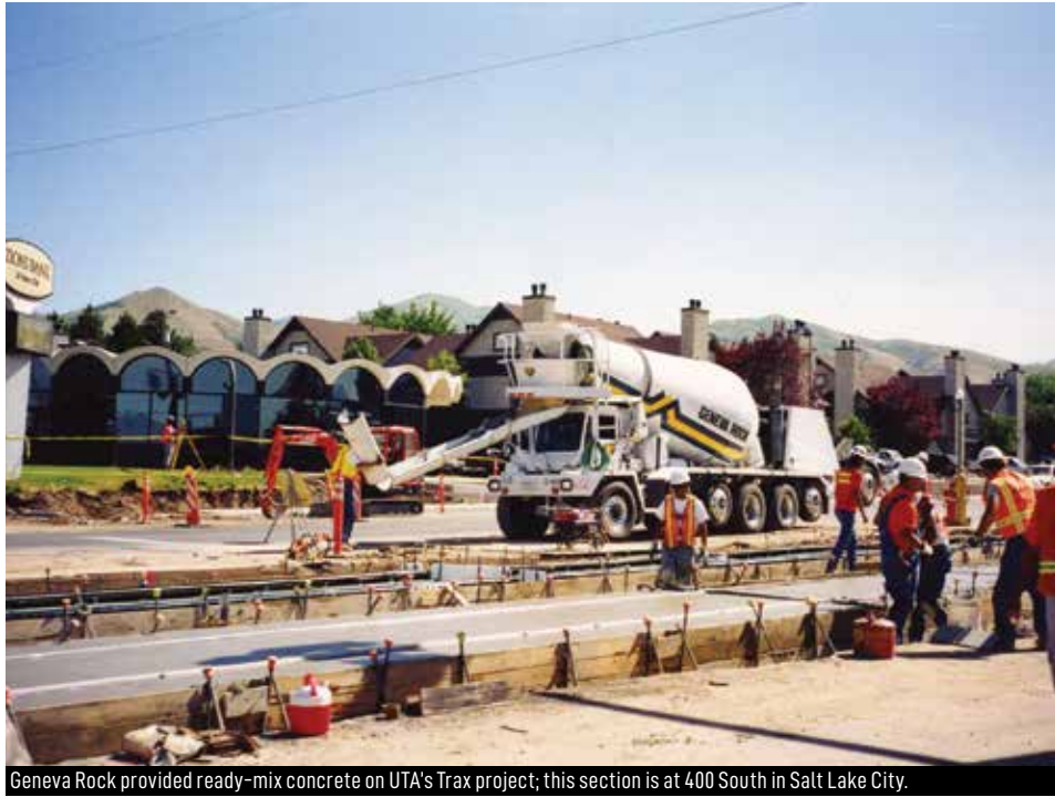
Geneva Rock provided ready-mix concrete on UTA’s Trax project; this section is at 400 South in Salt Lake City.
