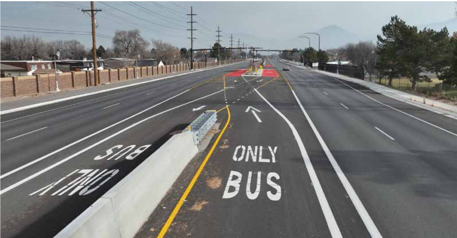
Doug Stremel, Sr. Project Manager with Jacobs, said extensive design work went into roadway geometry to ensure buses could navigate crossovers, like those pictured in the foreground, as they enter the boarding platforms in the background. (photo courtesy UTA)
