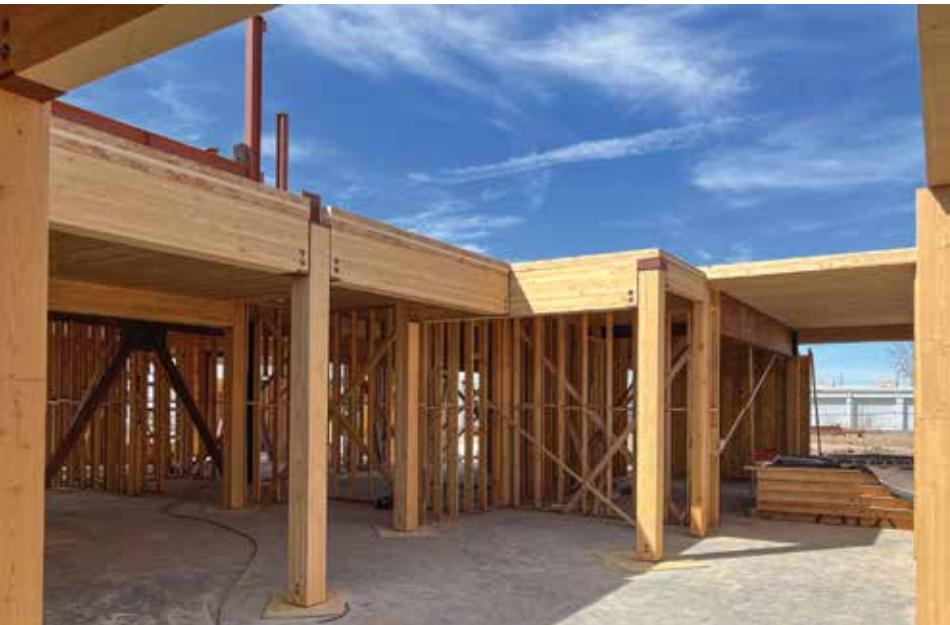
Timberwood Creek is a hybrid mass timber project designed by ASSIST and currently under construction led by KIER Construction. Its mass timber elements—CLT floor plates supported by glulam beams and columns—will deliver a biophilic living environment for the Davis Behavioral Health clients who will soon call it home. (top photo courtesy KIER; rendering below courtesy ASSIST)
