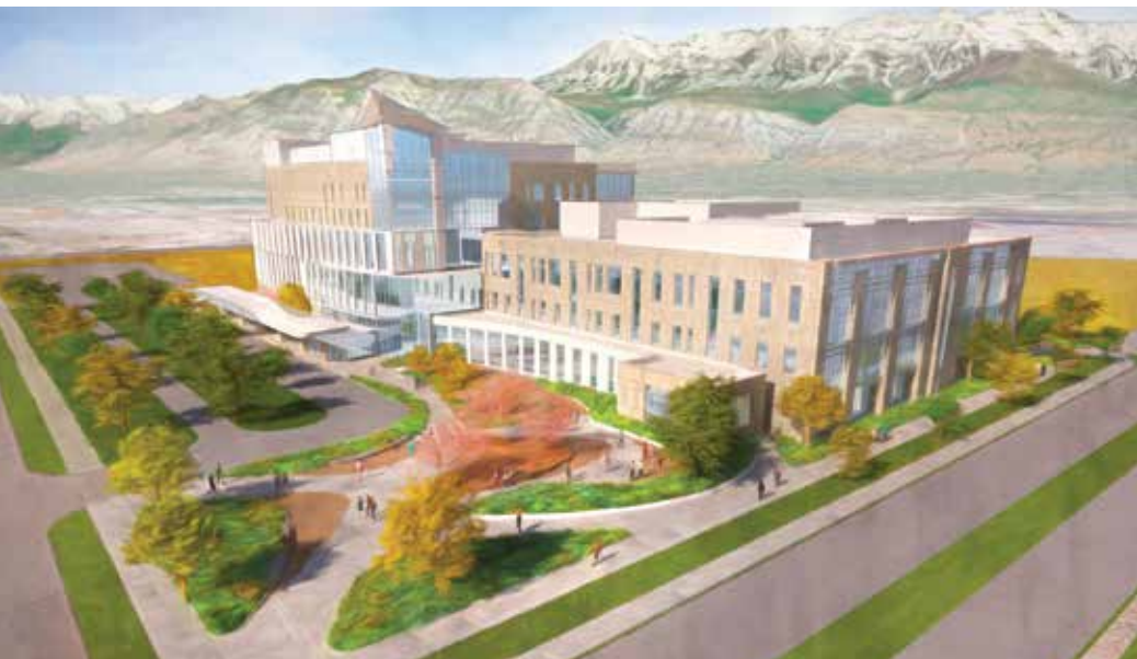
Rendering of Phase I of the Huntsman Cancer Institute's Comprehensive Cancer Center in Vineyard, which held a groundbreaking April 8. (courtesy Huntsman Cancer Institute, Architectural Nexus)
