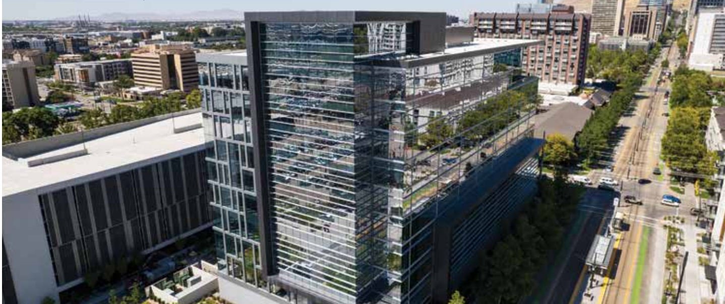
650 South Main Office - Salt Lake City
