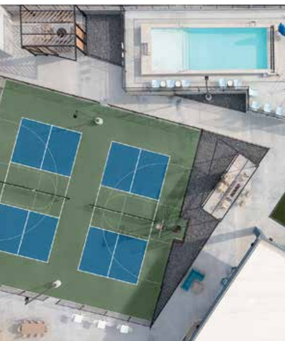
Amenity spaces at Seven02 Main Apartments at 702 S Main St. Salt Lake City, are designed to enhance recreation and work for tenants and play a vital role in maintaining strong occupancy. (photos courtesy PEG Companies)
