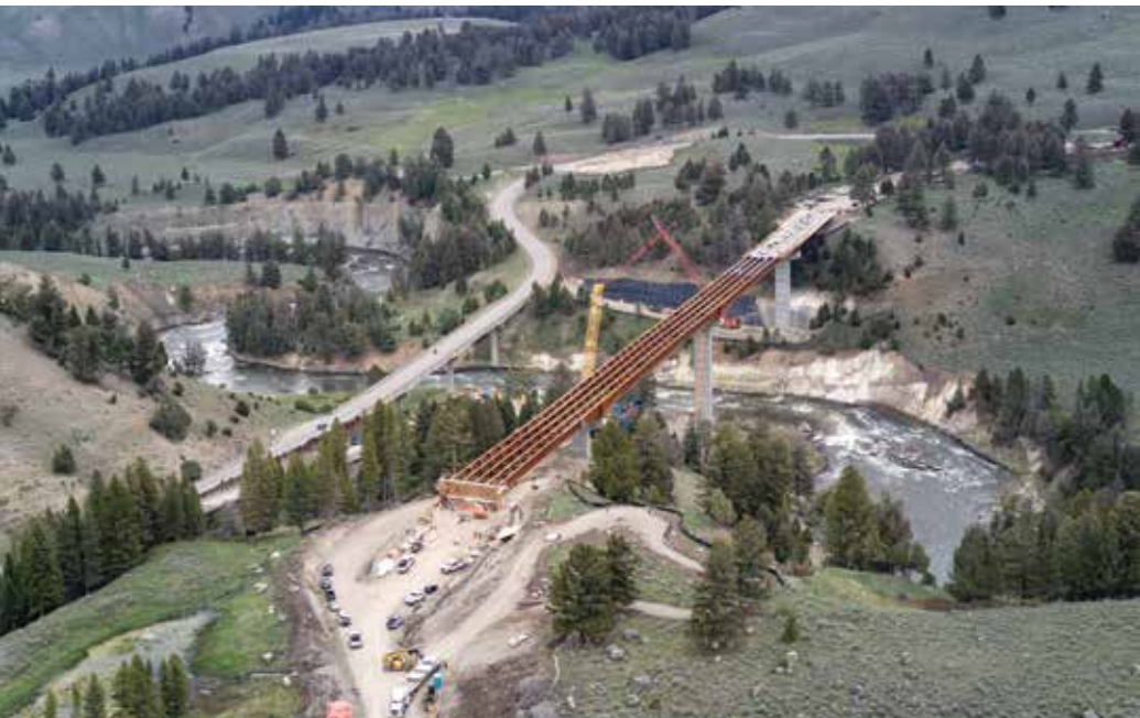
Bridge building remains RLW’s forte, including this complex replacement of the Yellowstone River Bridge located at Tower Junction (Wyoming). The project calls for the replacement of the 60-year-old bridge with a new, one-quarter mile (1,285-foot) steel girder bridge, along with realigning a mile of the Northeast Entrance Road.
