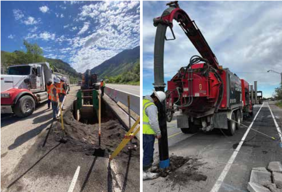
COP Construction completed its $9 million section of the Salt Lake Aqueduct/Cottonwoods Connection project last fall, installing over 6,500 feet of new 36-inch welded steel pipe between Big Cottonwood WTP and the existing aqueduct near Fort Union Blvd. (photos courtesy COP Construction)
