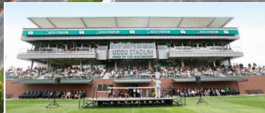
Aerial view of UCCU Stadium at UVU, an exciting addition to the school's athletics program. (inset) Front view of the bleachers, press box, and suites. (photos courtesy SIRQ Construction)
