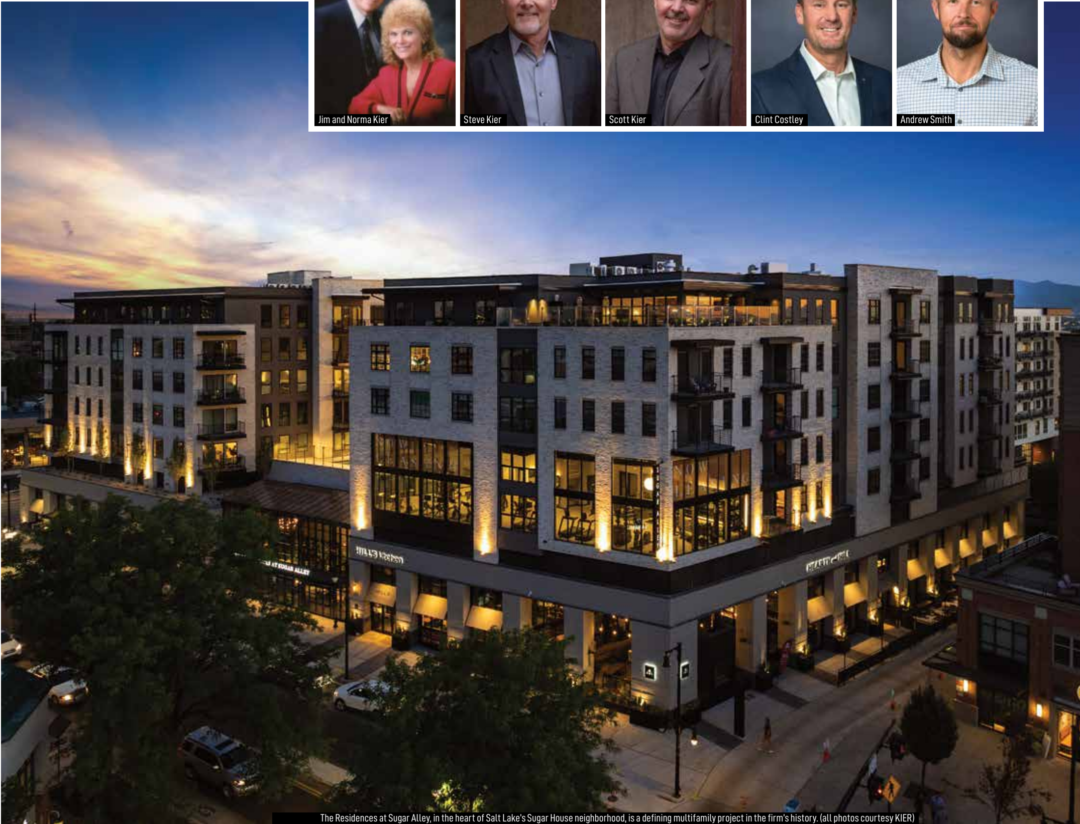
The Residences at Sugar Alley, in the heart of Salt Lake’s Sugar House neighborhood, is a defining multifamily project in the firm’s history. (all photos courtesy KIER)
