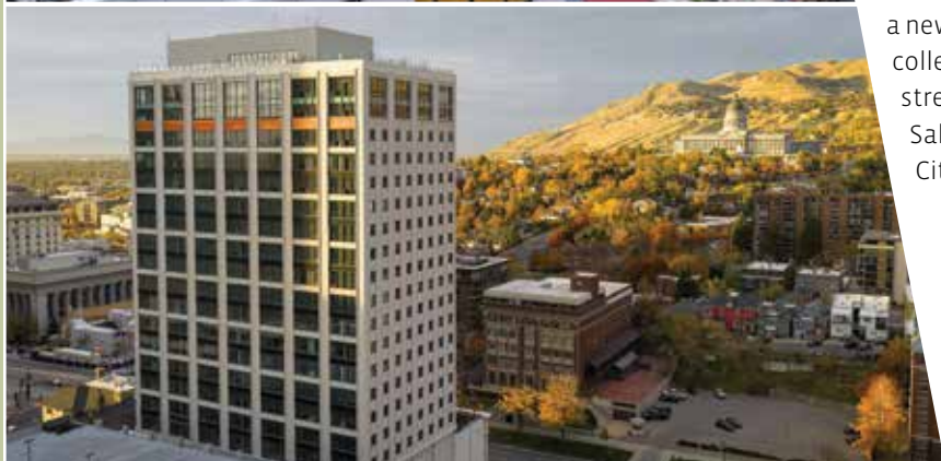
(Pictured) Seraph stands tall along the Salt Lake City skyline, with its new copper band sitting just below the penthouse floor, a crowning achievement for Utah's first adaptive reuse high-rise. The project delivered 217 luxury residences (top of image set), rooftop amenities (middle), and transformed the top floor of the existing parking garage into a mid-level amenity deck (image above project box). (photos by Hines; courtesy Big-D Construction)
