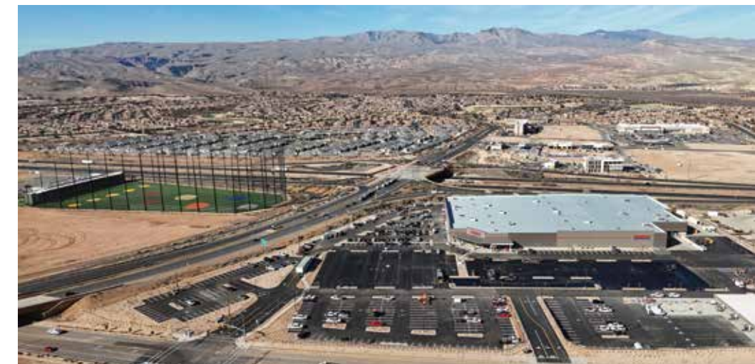
St. George saw the recent opening of its second Costco (right) at the south end of the city. Only a handful of cities nationwide (less than 150,000 people) can boast having more than one of the popular retail warehouses. (photo courtesy City of St. George)
