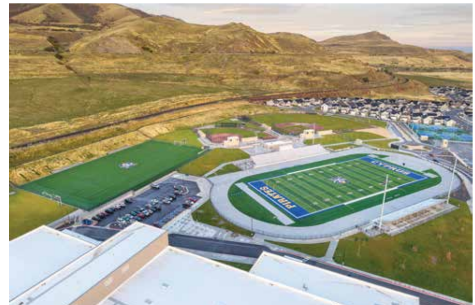
(pictured) The project team expertly navigated the project’s 57-acre site, building out a school and an impressive sports complex with views up to the Oquirrhos. (above) Views down to the auditorium stage showcase the project team’s impressive ability to design and deliver flexibility within massive volumes, where the expanded bleachers visible at the bottom of the image can be collapsed to make way for a sizable multi-use space for students and staff.
