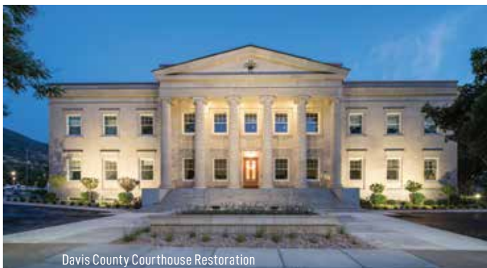
Davis County Courthouse Restoration
