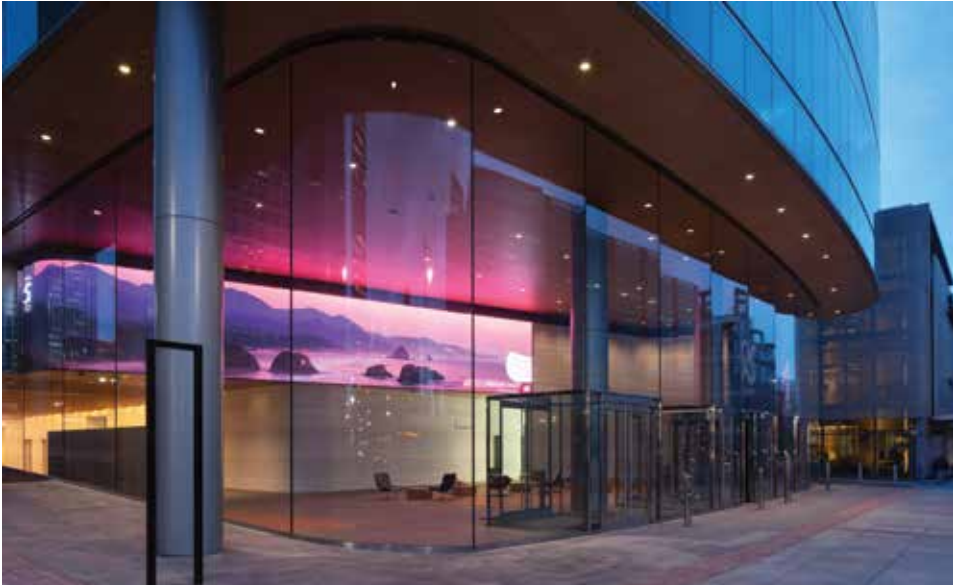
Steel Encounters has excelled in the fabrication and installation of all-glass curtain wall exterior systems in the past 15 years, including 95 State (left) in Salt Lake and the Nu Skin Innovation Center in Provo. Crews utilize specialized equipment with huge suction cups to lift huge pieces into place. (all photos courtesy Steel Encounters, except where indicated)
