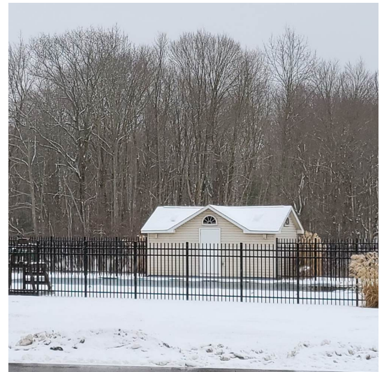
Thanks to a generous donation from Board Member, Alice Dalmaso, we were able to install a new fence around our now newly named Getty Pool.
