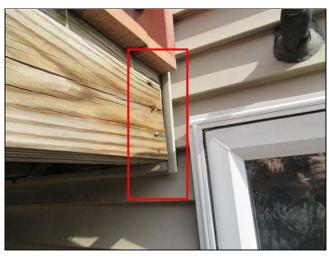
**2.6** (5) There was a hole under the lattice at the front porch. There is a potential for critters to get under the porch. I recommend that the holes be filled back in.
