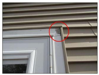
**2.0** (2) There was a gap where the AC refrigerant line penetrated through the wall of the house. This gap will reduce the energy efficiency of the house and could potentially allow insects access in to the house. I recommend that this gap be properly sealed.
