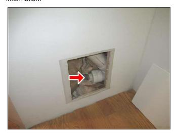
**6.4** (2) The pop-up did not operate in the third floor bathroom tub. There is no way to hold water in the fixture with this pop-up. I recommend that a licensed plumber repair or replace the pop-up.
