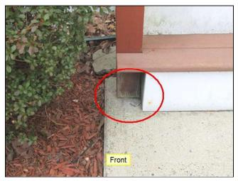
**2.6** (4) The perimeter joist on the right side of the rear deck was split and pulling away from the ledger board due to inadequate fasteners. One nail, at the split, could be pulled out by hand. This can threaten the structural integrity of the deck. I recommend that a qualified contractor replace the spilt rim joist and use the appropriate mechanical fasteners to secure it to the ledger board.
